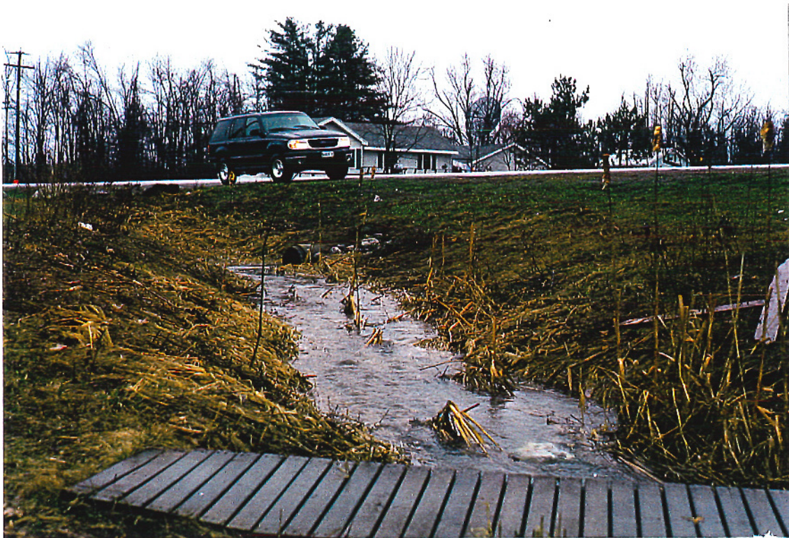
HEAD OF LAKE STREAM- Intermittent stream with cloudy water with obvious sand delta in lake . Drainage is from a 20 acre field that is well vegetated with stable soil. Small wet land present on upland side of culvert. Silt fencing or more permanent structure may help. Priority Medium. Site B 2 Photos
