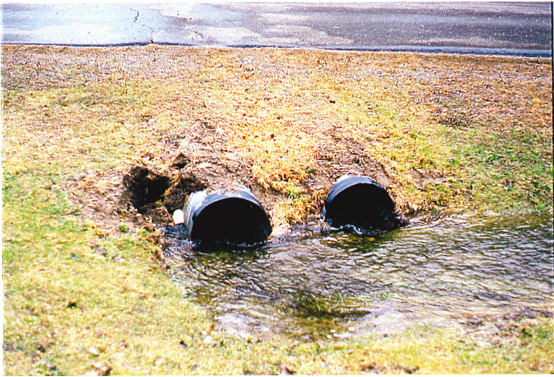
Eroding culverts on the upper portion of Parmenter Drive
