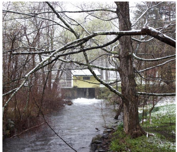
The outlet dam on Outlet Stream. (Photo Credit: Elaine Philbrook, CLA)
