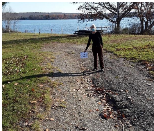
Roads and driveways built to access new development can deliver large quantities of sediment and attached P if not built correctly or maintained properly. (Photo Credit: CLA)
